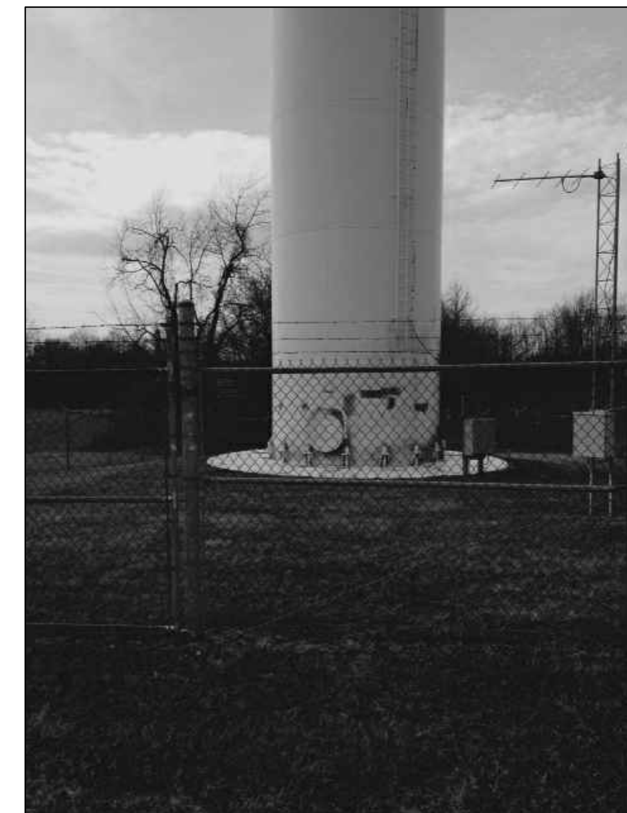
GROUND VIEW - KINGS RIDGE TANK
